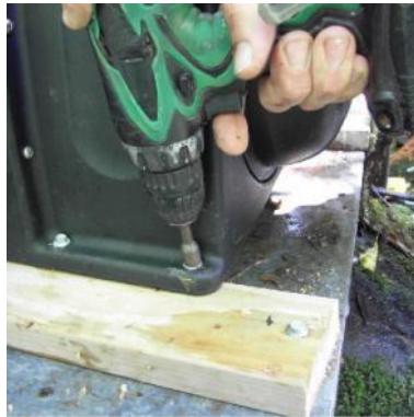
Fixing a turbine to a timber base
